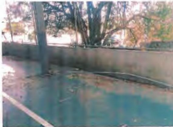
Figura 11: Recalque do piso
